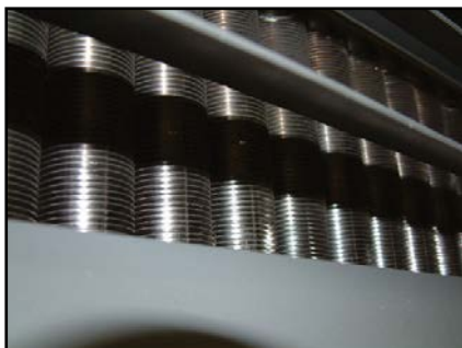
Liquid-to-air heat exchanger
